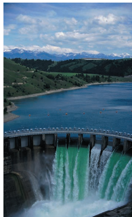
FIGURE 3-10 Potential and Kinetic Energy Water stored behind a dam has potential energy. The water flowing over the spillway has kinetic energy.
