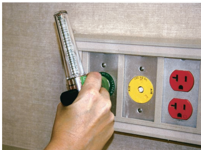
Figure 50–10 ■ Insert flow meter into the wall unit.
