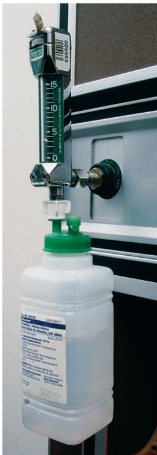
Figure 50–9 ■ An oxygen humidifier attached to a wall outlet oxygen flow meter.
